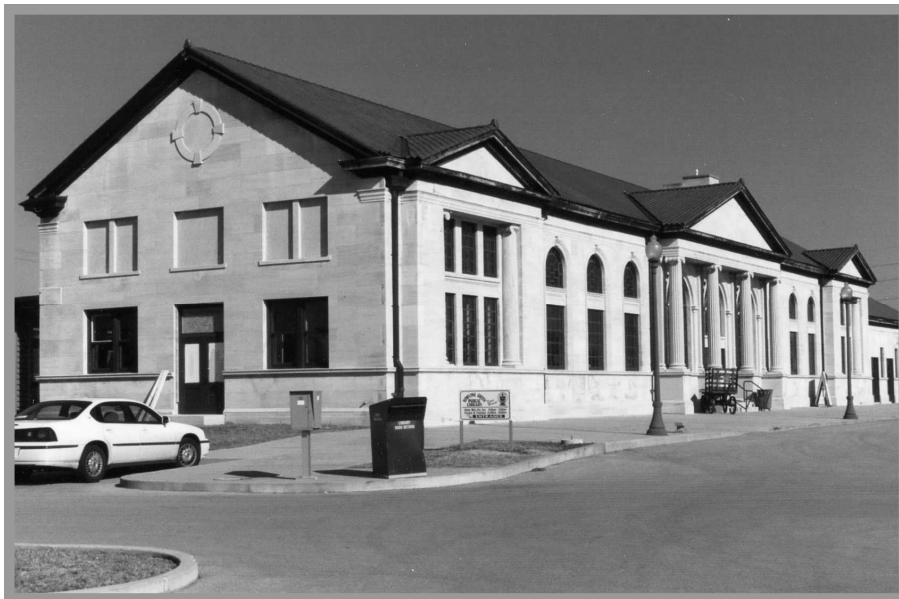
The old L&N passenger station at Bowling Green, Kentucky is in the process of a complete restoration and use as both a public library and a Museum. There are several vintage L&N passenger cars on the property. It's a shame we can't get Amtrak back in Central Kentucky. from a color print by Wallace
